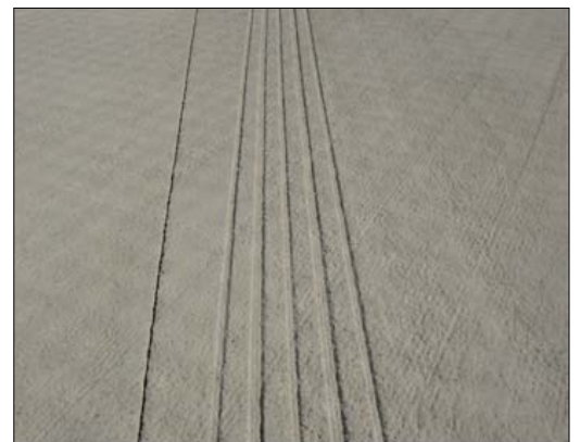
FIGURE 2 & 3 Grooved rooftop surface - drainage solution
