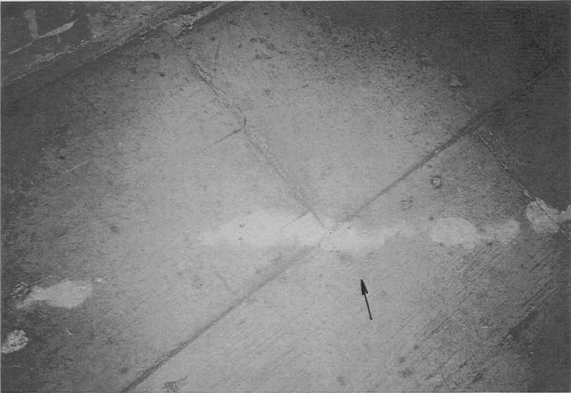
Photograph 20: View of soffit under pond before test.
