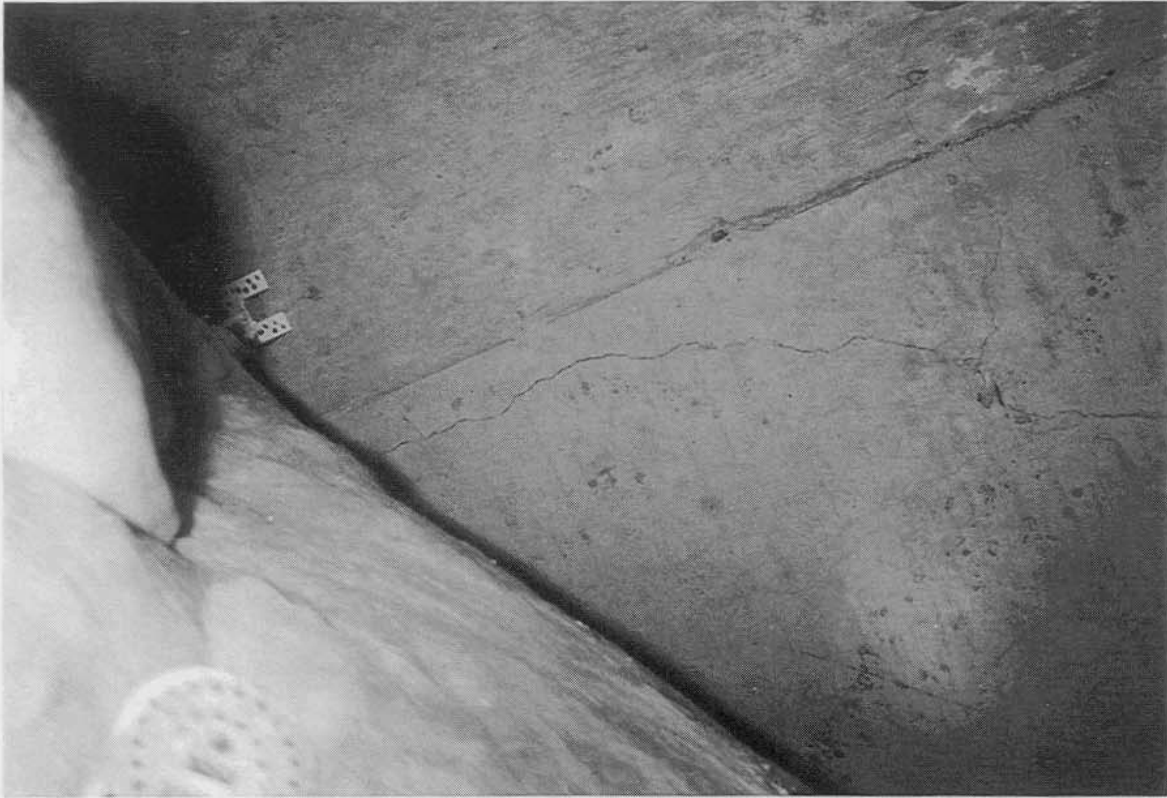
Photograph 8: View of soffit after ponding test, (30 mins)
