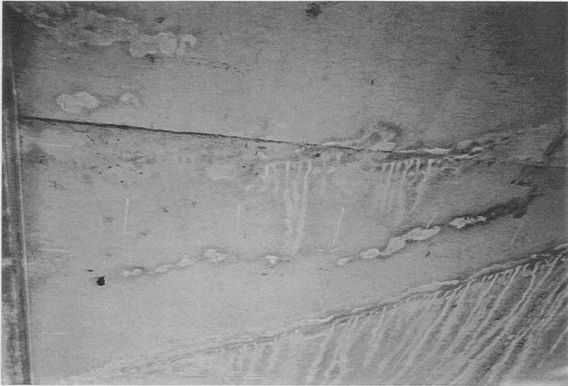
Photograph 2: View of soffit before ponding test
