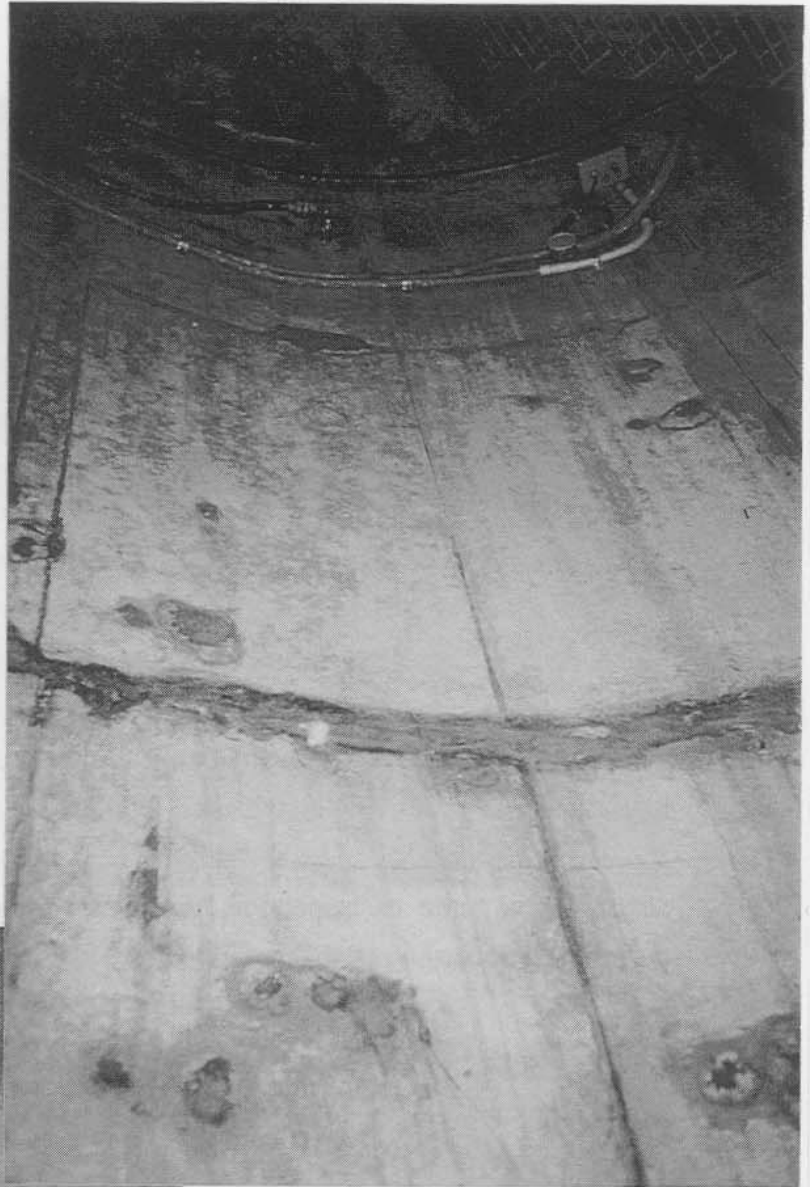
Photograph 14: View of construction joints from inside tower.
