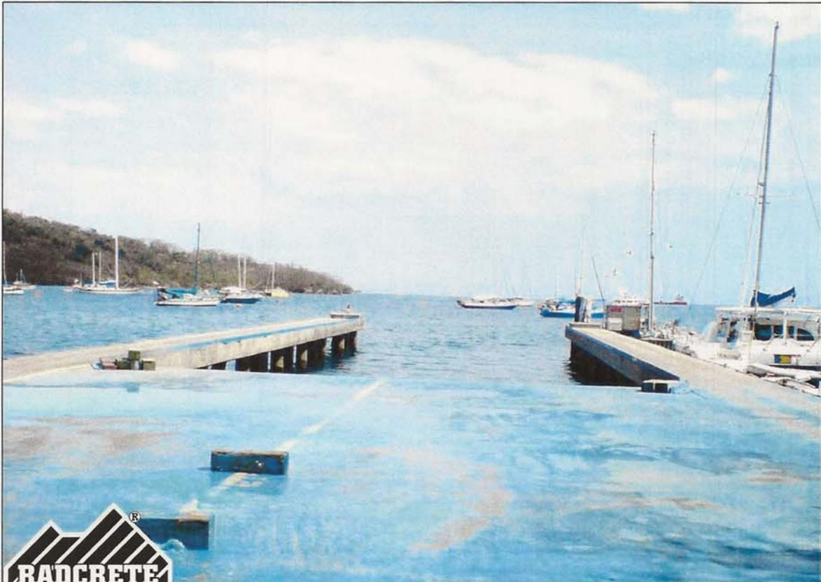
This marina was waterproofed with one of our competitor's products which failed after 3 years resulting in chloride ion attack. Dover was asked to repair the both top and underside of the marina. The slabs were sandblasted to remove any previous products, barnacles, etc. All areas were then washed with fresh water and treated with RADCON Formula #7, providing watertight seal and steel reinforcement protection to date.
