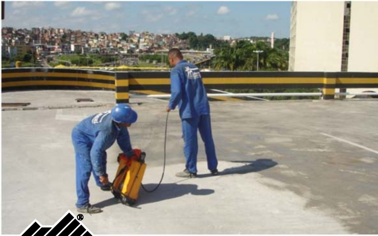
FIGURE 1-2. Radcon #7 spray-application on the rooftop car park.
