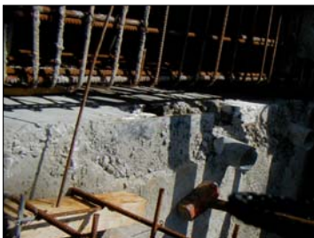
FIGURE 12. The reinforcement works
