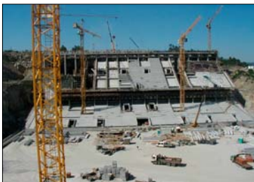
FIGURE 6. Progress in the construction works
