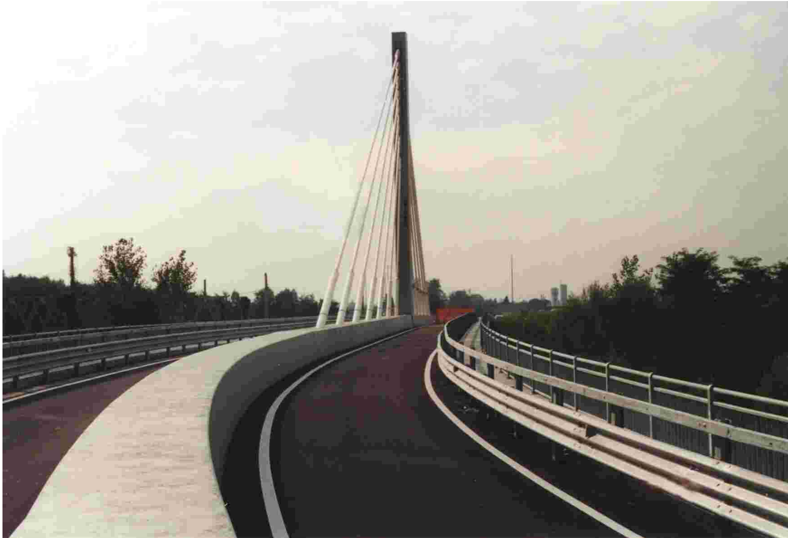
Bridge over Livenza river, (TREVISO) - 1.600 Sqm Waterproofing with RADCON #7 of the bridge deck.
