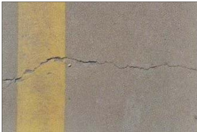
FIGURE 16. Close-up of one of the many cracks in the deck
