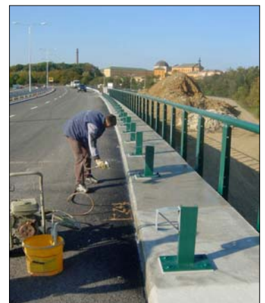
FIGURE 18. Radcon application using a diesel sprayer
