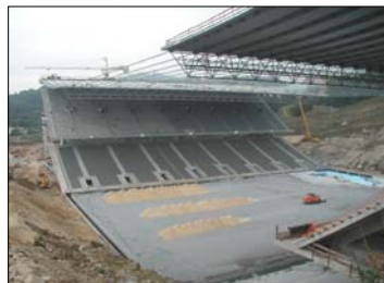
FIGURE 7. Steel connectors completed
