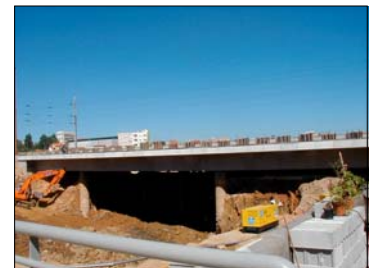
FIGURE 14. Works on Gaia Bridge
