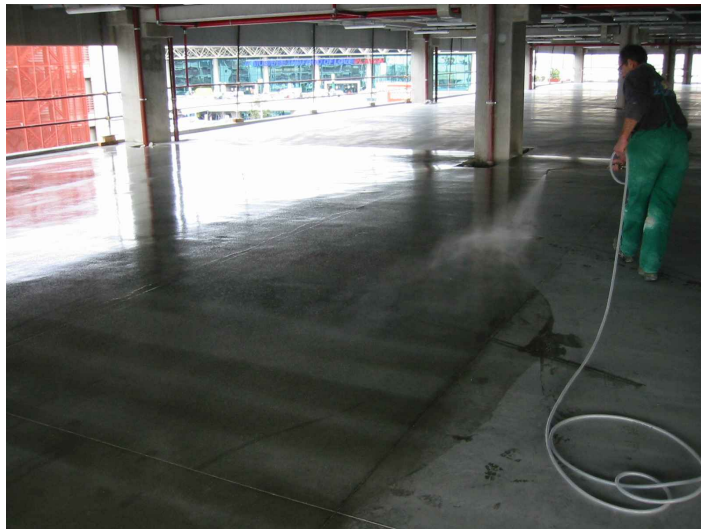
New parking "Fiumicino airport", ROMA - 35.000 Smq Waterproofing with Radcon #7 of the rooftop and the other parking level.
