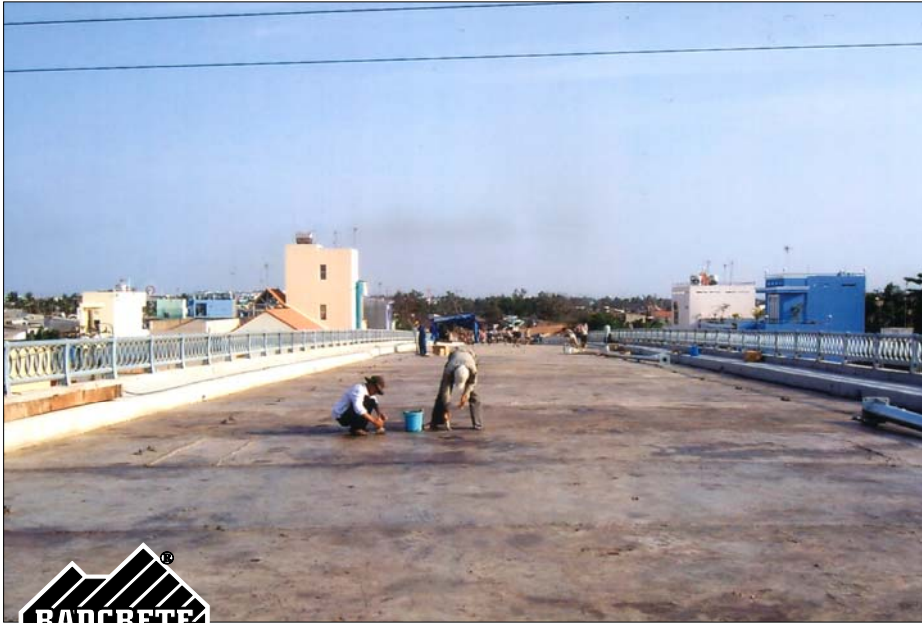
FIGURE 3. Kenh Te Bridge surface preparation prior to Radcon Formula # 7 application
