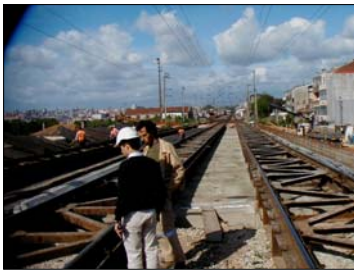
FIGURE 11. Inspecting the structure before waterproofing
