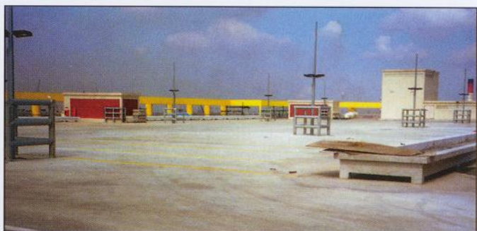
JTC FACTORY ROOF CAR PARK, RADCON#7 AND RADFLOOR TREATMENT, SINGAPORE
