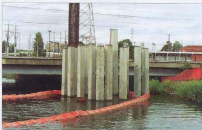
FIGURE 39 - PILES DRIVEN INTO MOONEE PONDS CREEK
