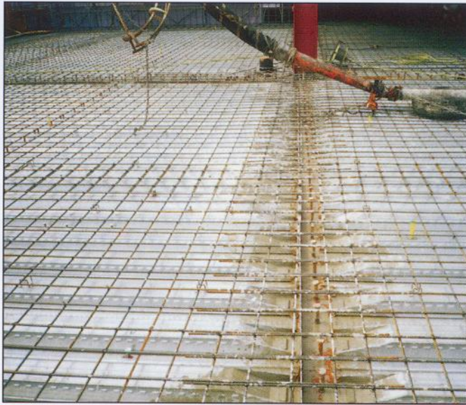
CONSTRUCTION USING STEEL PAN
