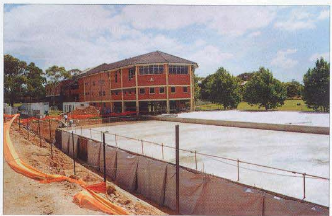
FIGURE 39 - SPORTSFIELD UNDER CONSTRUCTION
