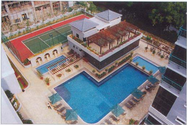
FIGURE 37 - RADCON #7 WATERPROOFS ENTIRE PODIUM LEVEL INCLUDING POOL, DECK, CLUB HOUSE AND TENNIS COURT
