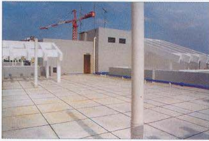
FIGURE 35 - INSULATION AND TOPPING OVER RADCON #7
