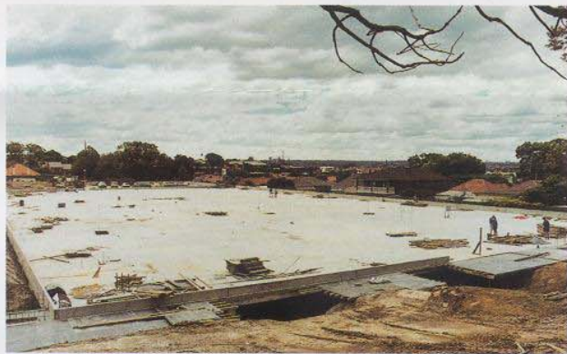
PHOTO 5 - SUSPENDED SLAB DURING CONSTRUCTION
