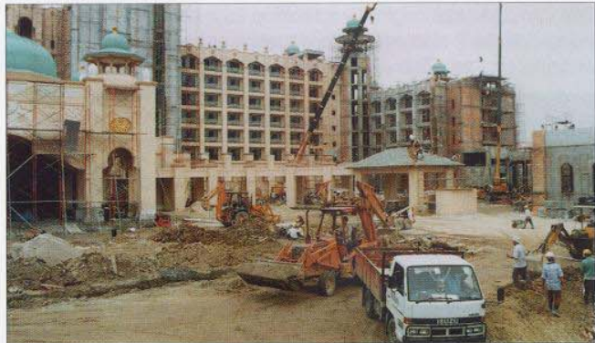
FIGURE 19 - BUSY SUSPENDED ENTRANCE AREA DURING CONSTRUCTION
