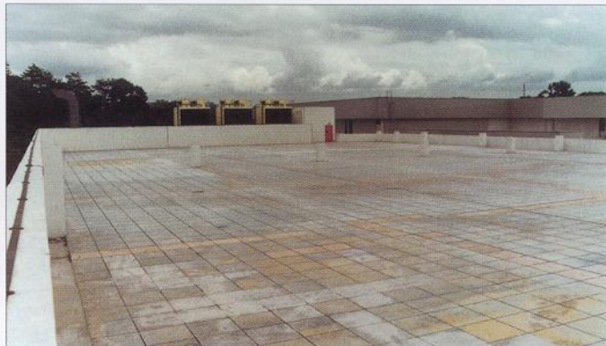
FIGURE 22 - ROOFTOP WITH TOPPING OVER RADCON #7 TREATMENT
