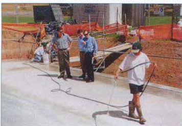
FIGURE 38 - RADCON #7 APPLICATION
