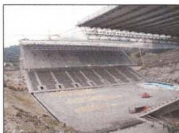
FIGURE 7. Steel connectors completed
