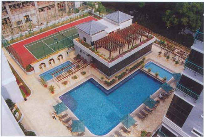
FIGURE 37 - RADCON #7 WATERPROOFS ENTIRE PODIUM LEVEL INCLUDING POOL, DECK, CLUB HOUSE AND TENNIS COURT
