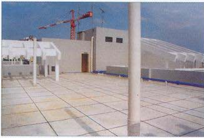
FIGURE 35 - INSULATION AND TOPPING OVER RADCON #7
