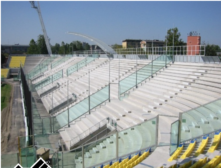
FIGURE 1. RADCON #7 treated stands.
