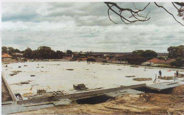
PHOTO 5 - SUSPENDED SLAB DURING CONSTRUCTION
