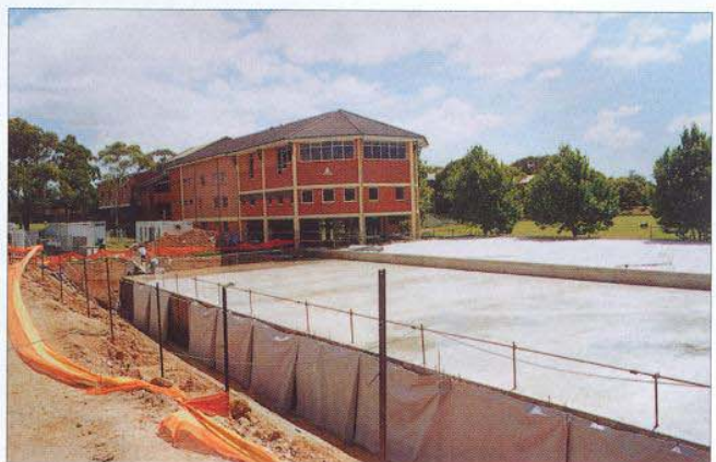
FIGURE 39 - SPORTSFIELD UNDER CONSTRUCTION
