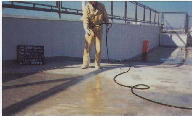
FIGURE 35 - RADCON #7 APPLICATION
