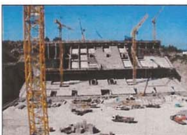
FIGURE 6. Progress in the construction works
