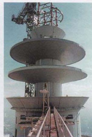
PHOTO 7 - LEVELS 9 & 10 OF THE TOWER HEAD
