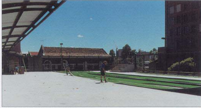
FIGURE 32 - ARTIFICIAL TURF LAID OVER RADCON #7
