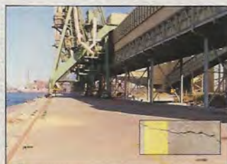
Grain Berth, Port Kembla, Wollongong, Australia. Radcon #7 alone, was used to seal these leaking cracks up to 2.00mm.
