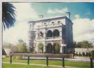
Heritage Building, Melbourne, Australia. This single skinned rendered building had leaked through the facade for many years. After several coats of paint were removed Radcon #7 was applied to stop all leakage.
